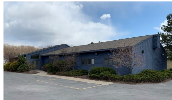
VIEW OF ADJACENT(REAR) SPACE AND MAIN ENTRANCE FROM PARKING LOT
